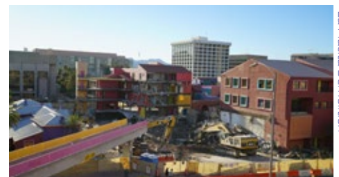
La Placita Demolition
